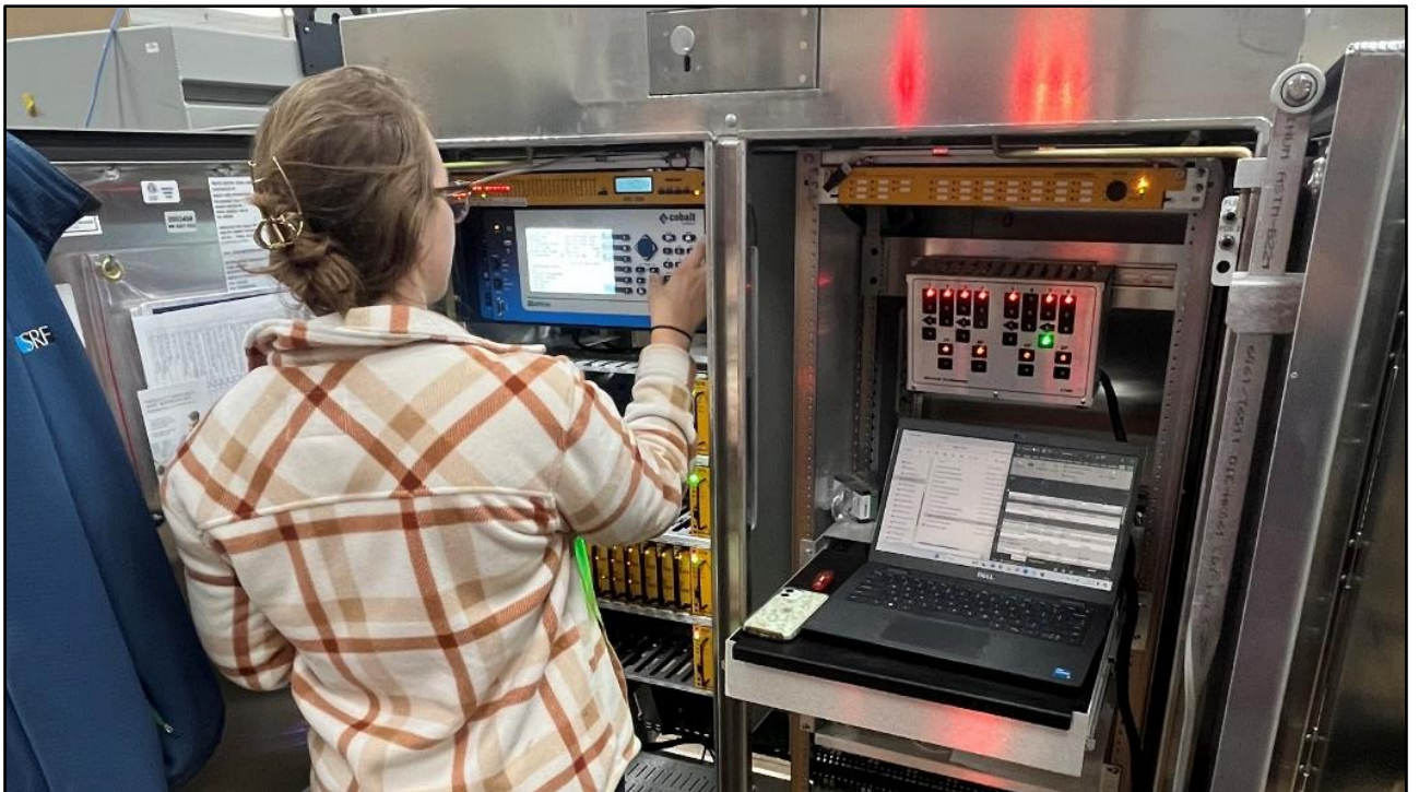
Stage 4 Testing, Cabinet Testing (SRF Consulting)
